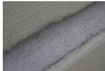
2. Fillet installed with KÖSTER Repair Mortar
