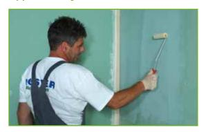
KÖSTER BD 50 Primer is applied to the substrate by roller or brush. Different substrates require different consumptions of the KÖSTER BD Primer. For priming gypsum board, dilute KÖSTER BD 50 Primer with water in a ratio of 1:3. Consumption of that mixture is approx. 240 g/m². For details on other substrates, refer to the technical data sheet of KÖSTER BD 50 Primer.
