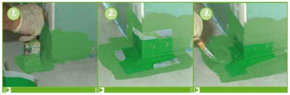
Apply a covering coat of KÖSTER BD 50 to the area on the outside corner where the KÖSTER BD Outside corner is going to be installed approx 10 cm up onto the wall and 10 cm onto the floor.
