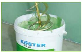
The first step is to stir up KÖSTER BD 50. Use a slowly rotating electrical mixer (400 rpm) to stir the material in the bucket for 1 minute.
