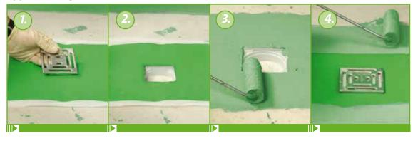
Position the KÖSTER Floor Sleeve over the floor drain on which it is applied. Cut a hole of the shape of the opening of the inside area of the floor drain into the KÖSTER BD Floor Sleeve. The hole should be smaller than the drain so that it overlaps approx. 3 mm. Apply a covering coat of KÖSTER BD 50 to the area around the floor drain where the KÖSTER BD Floor Sleeve is going to be installed.
