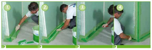
Apply a covering coat of KÖSTER BD 50 to the area where the KÖSTER BD Flex Tape K 120 is going to be installed.
