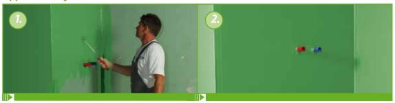
KÖSTER BD 50 is applied to the area using a roller or a brush. Application of waterproofings is always done in at least 2 coats. Consumption per coat is approx. 0.5 to 0.6 kg /  $m^2$  leading to a total consumption of approx. 1.1 kg /  $m^2$ . Waiting time between coats is at least 3 hours.
