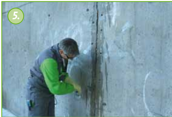
Pre-wet the crack
