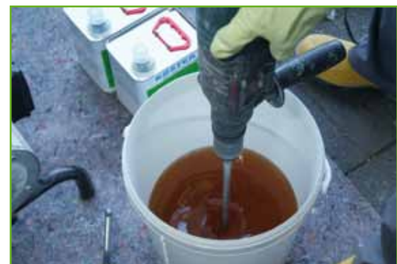
A suited stirrer such as the KÖSTER Resin Stirrer in combination with a slow rotating mechanical mixing device is used to mix both components. The components are mixed until the material is homogenous.
