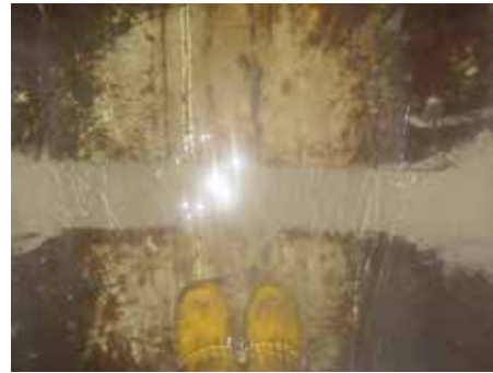
Very stable - even under flowing water
