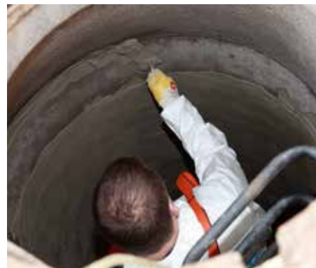
Connection of the shaft to the entrance area
