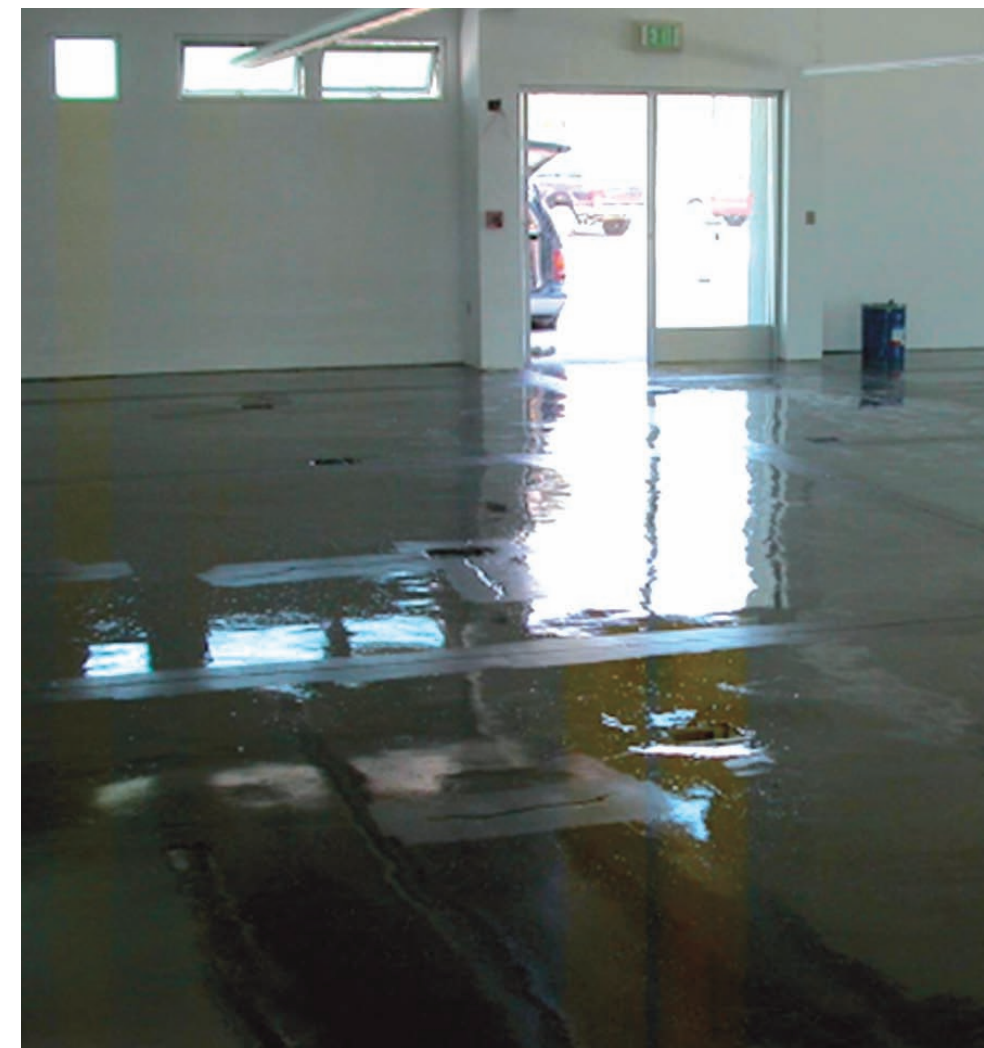
Finished VAP-I® 2000 Project
