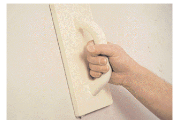
... and – once it has just started to set – leveled with a trowel
