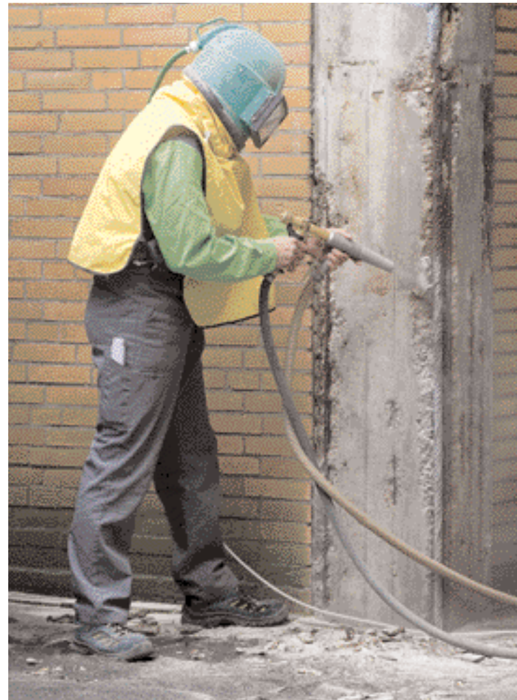
Cleaning the steel reinforcement and concrete by sand-blasting
