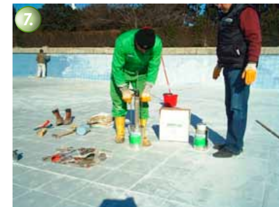
The joints also have to be implemented in the tiles.
