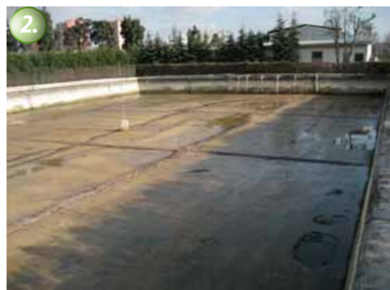
The surface is cleaned down to a solid and stable base material. The substrate must be clean, solid, and free from adhesion inhibiting materials.
