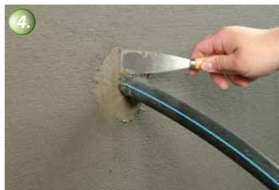
The pipe penetration is now permanently waterproofed.
