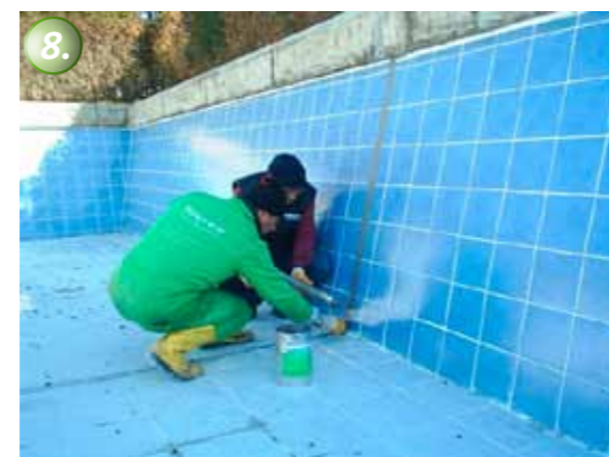
The horizontal joints are waterproofed with KÖSTER Joint Sealant FS-H. The vertical joints were waterproofed with the putty-like KÖSTER Joint Sealant FS-V.
