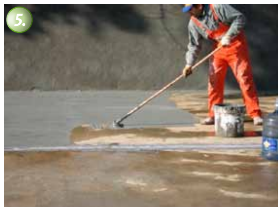
5. The area waterproofing is done with KÖSTER NB 1 Grey.
