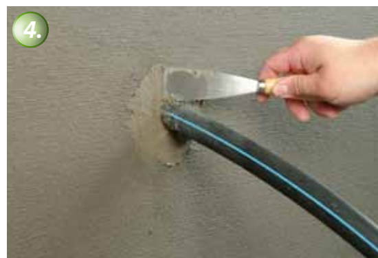
The pipe penetration is now permanently waterproofed.
