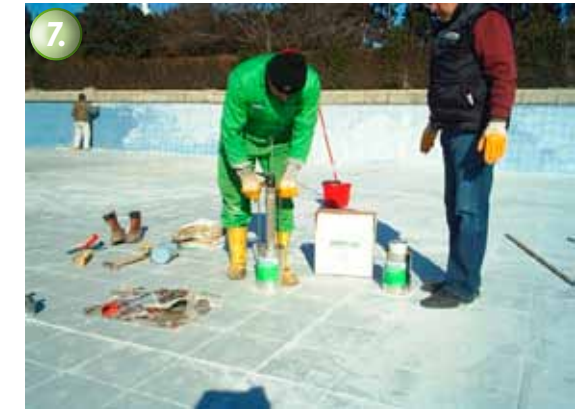
7. The joints also have to be implemented in the tiles.
