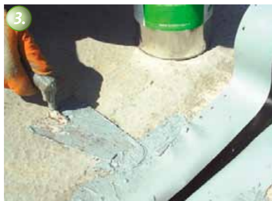
To give the KÖSTER Joint Tape more tolerance, it is pressed slightly into the joint.
