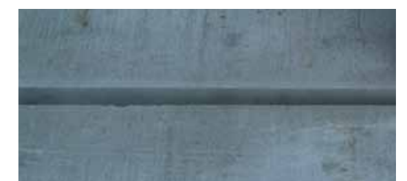
Cleaned joint flanks
