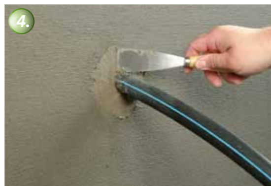
The pipe penetration is now permanently waterproofed.
