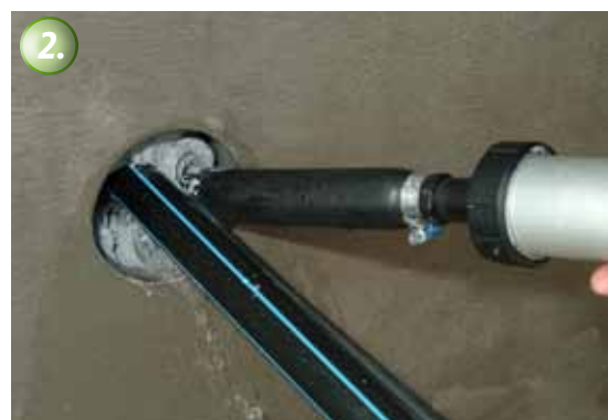
The material is pressed into place between the cable and the wall with the KÖSTER Special Caulking Gun, immediately and permanently stopping the water flow.
