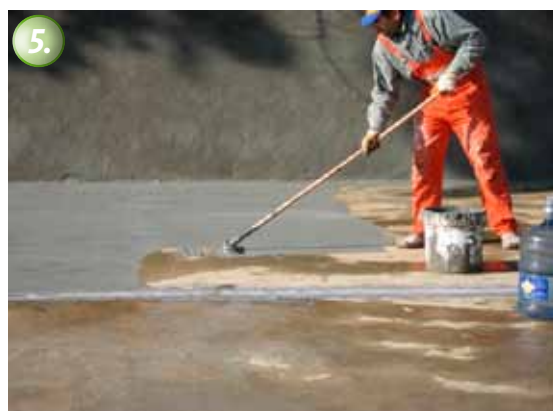
The area waterproofing is done with KÖSTER NB 1 Grey.
