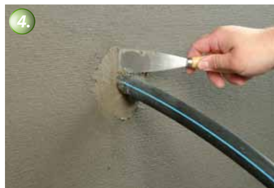
The pipe penetration is now permanently waterproofed.
