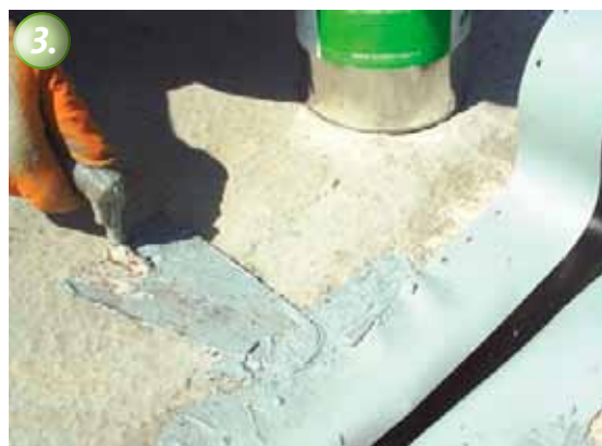
3. To give the KÖSTER Joint Tape more tolerance, it is pressed slightly into the joint.
