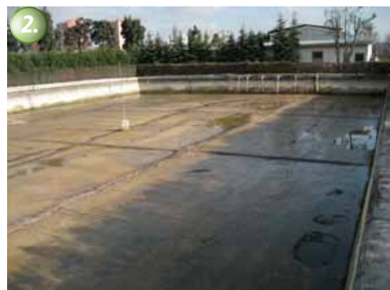
2. The surface is cleaned down to a solid and stable base material. The substrate must be clean, solid, and free from adhesion inhibiting materials.
