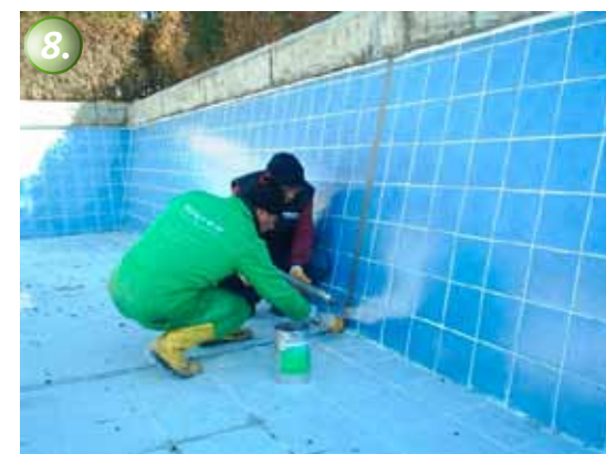
8. The horizontal joints are waterproofed with KÖSTER Joint Sealant FS-H. The vertical joints were waterproofed with the putty-like KÖSTER Joint Sealant FS-V.
