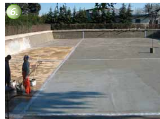
6. The tiles are applied on top of the waterproofing with common tile adhesive.
