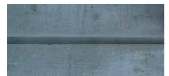
Cleaned joint flanks
