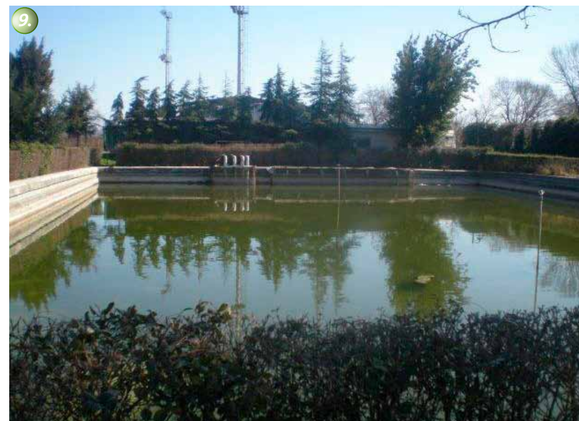
9. The KÖSTER joint and area waterproofing system has proved itself for years at the Veli Efendi Racetrack and still reliably serves the basin as an unfailing waterproofing.
