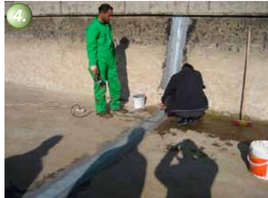
Connections are made with a hot air welding gun; seams should overlap at least 2 cm.
