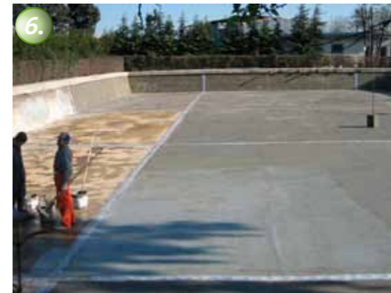
The tiles are applied on top of the waterproofing with common tile adhesive.
