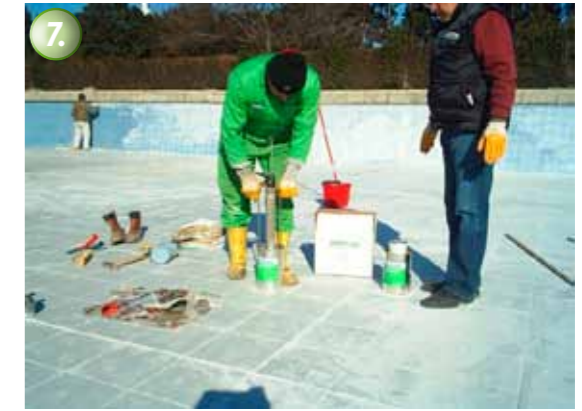
The joints also have to be implemented in the tiles.
