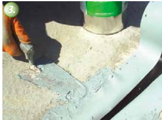
To give the KÖSTER Joint Tape more tolerance, it is pressed slightly into the joint.
