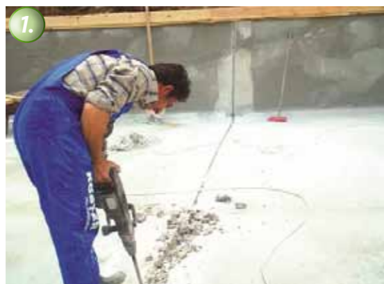
The debris and remnants of the concreting work are removed.
