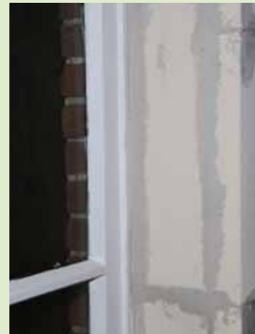
boards are also available. These are applied flush to the previously installed wall boards and offer an optimal finish.
