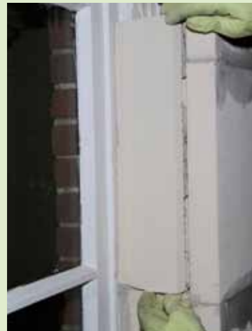
For detailed areas such as jambs and soffits around windows and doors that won't allow using the 50 mm thick boards, 25 mm
