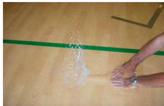
...containing high pH corrosive liquid
