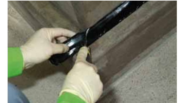
Fillets can be made of either KÖSTER Repair Mortar or alternatively with the cold self-adhesive KÖSTER KSK Triangular Ribbon.
