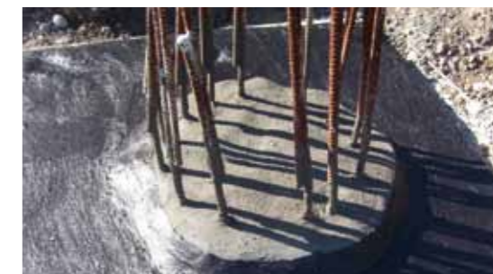
Connection of the area waterproofing (KÖSTER Deuxan®) to the pile head waterproofing
