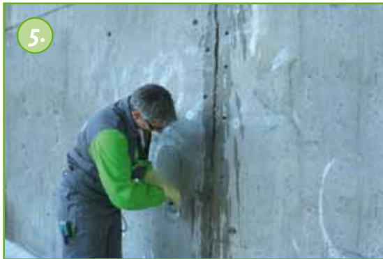
Pre-wet the crack
