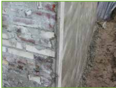
2. The substrate can be dry or slightly moist. Repair damaged areas as well as cracks and holes with KÖSTER WP Mortar.
