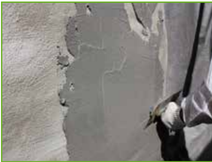
4. Apply the first coat by flat trowel, tooth trowel, or appropriate spray equipment.
