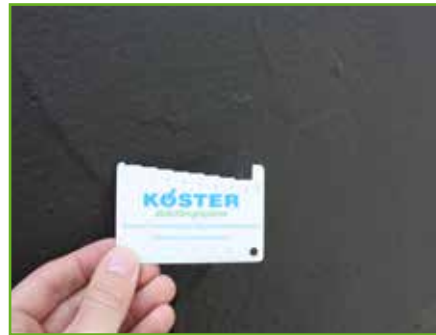
6. KÖSTER NB 4000 waterproofing is safe and easy. Backfilling permitted after approx. 24 hours.
