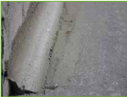
1. Corners are rounded out with a fillet made from KÖSTER WP Mortar.
