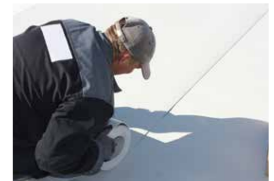
The membrane is positioned and then welded.
