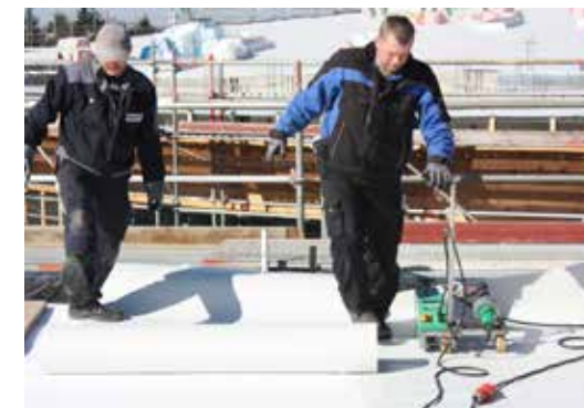
The KÖSTER TPO Membrane is unrolled.
