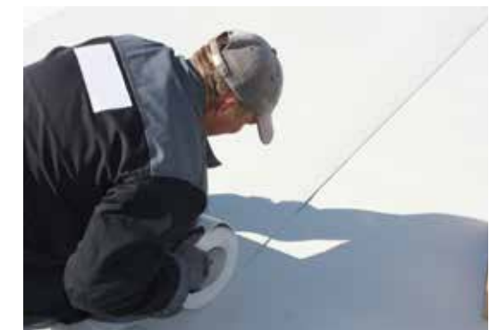
The membrane is positioned and then welded.
