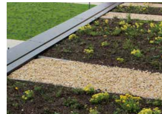
A greened flat roof with low vegetation. The individual flowerbeds are lined with gravel.
