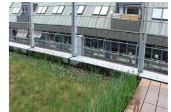
A greened and accessible flat roof with medium-high vegetation adjoined to a wooden terrace.
