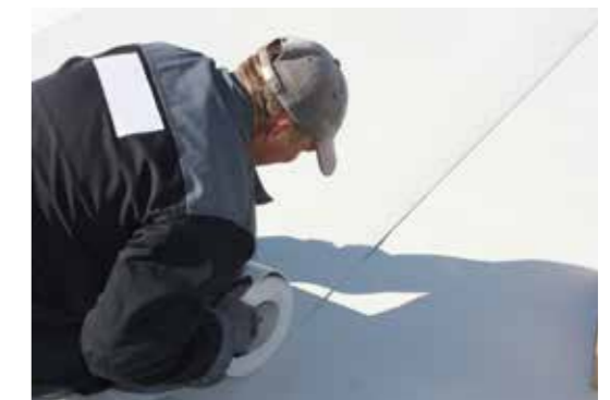
The membrane is positioned and then welded.
