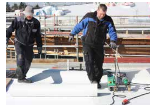
The KÖSTER TPO Membrane is unrolled.
