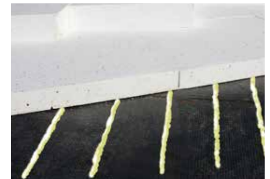
Next, the insulation is adhered. It is recommended to use KÖSTER PUR Membrane Adhesive.
