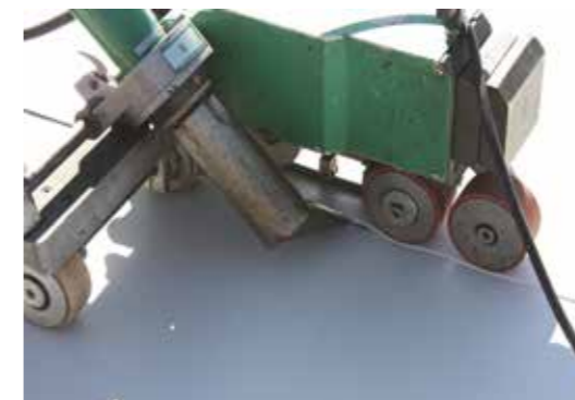
A welding machine simultaneously performs the tasks of pre-fixing, heating, and pressing, creating a homogenous bond among the membranes.
