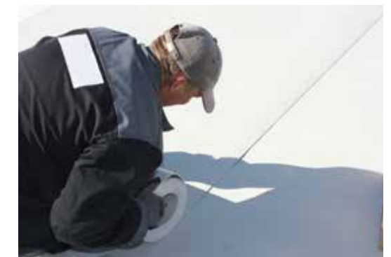
The membrane is positioned and then welded.
