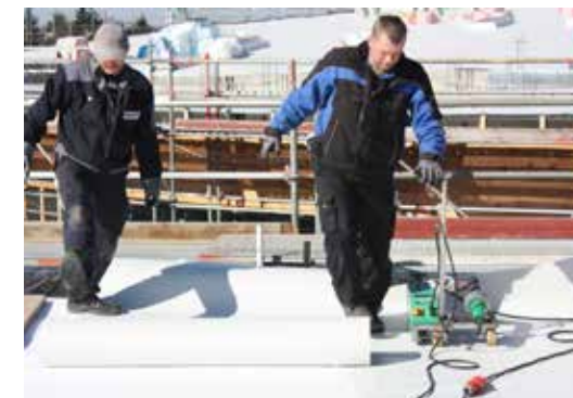
The KÖSTER TPO Membrane is unrolled.
