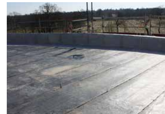
Preparation of a roof surface. A vapor barrier is used as the basis for further installation.
