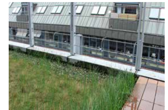
A greened and accessible flat roof with medium-high vegetation adjoined to a wooden terrace.
