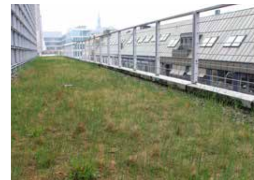
A greened and accessible flat roof with grass and vegetation.
