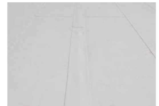
Additional mechanical fastening centered in the membrane may be necessary in order to protect the TPO membrane against high loads.
