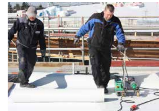
The KÖSTER TPO Membrane is unrolled.
