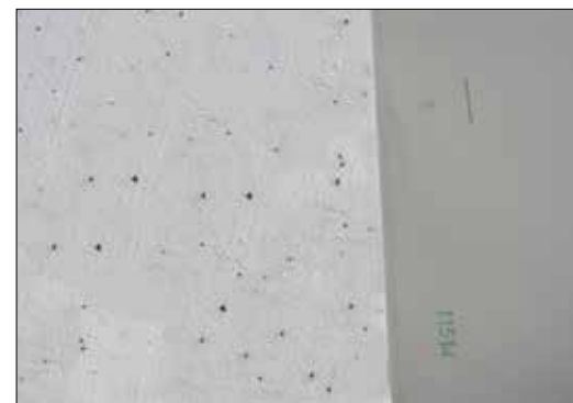
Direct installation over EPS insulation
