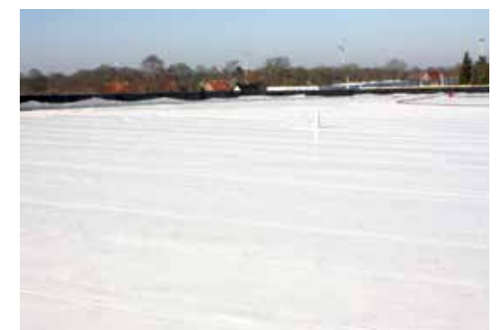
After welding all seams, the selected ballast can be installed.
