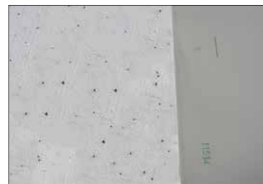
Direct installation over EPS insulation
