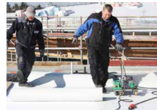
The KÖSTER TPO Membrane is unrolled.
