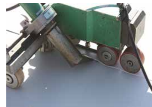
A welding machine simultaneously performs the tasks of pre-fixing, heating, and pressing, creating a homogenous bond among the membranes.
