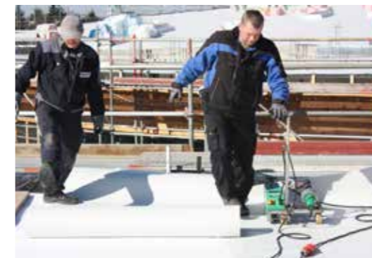
The KÖSTER TPO Membrane is unrolled.
