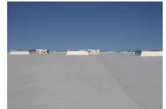
KÖSTER TPO Membranes are connected to individual SHEV-flaps with KÖSTER Contact Adhesive.
