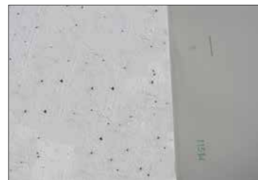
Direct installation over EPS insulation
