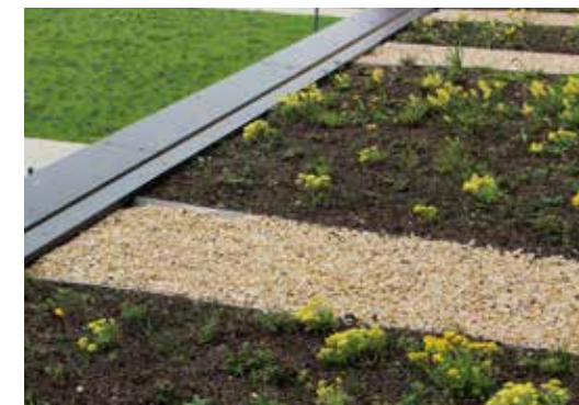
A greened flat roof with low vegetation. The individual flowerbeds are lined with gravel.
