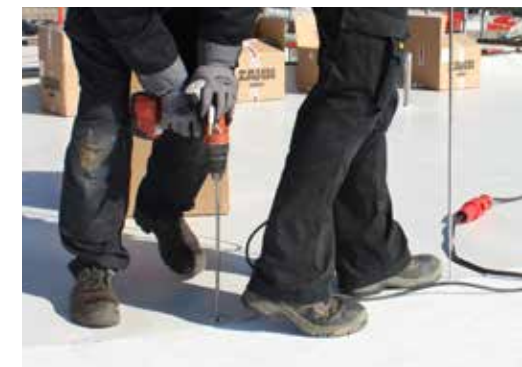
The KÖSTER TPO Membrane is mechanically fastened by attaching the disc anchors to the substructure. In this case, trapezoidal sheet metal.
