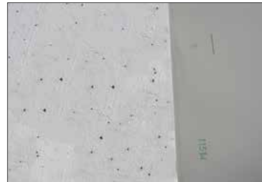
Direct installation over EPS insulation
