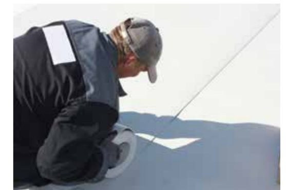
The membrane is positioned and then welded.
