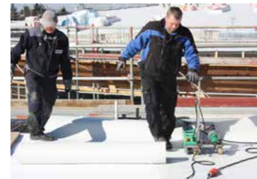
The KÖSTER TPO Membrane is unrolled.
