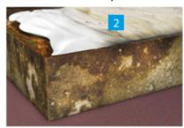
operations begin. This phase uses hot water and a deck spinner washer to clean the surface from the oil that has been washed out and the remaining foam. After the rinse a squeegee and a vacuum is used to remove all standing water from the area to be coated. Depending on the level of contamination more KÖSTER ORS-D treatments can be necessary.
