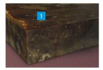
substrate must be sound and absorptive and should furthermore be free of Alkaline Silica Reactive or sulphurous compunds. Any type of surface contamination such as adhesives, adhesive residue, old coatings, curing compounds and underlayments must be removed completely by shot blasting prior to the ORS treatment being applied.
