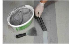
Remove the black masking tape while the adhesive is fresh.
