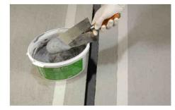
Mix the A and B components of KÖSTER KB-Pox Adhesive as stated in the technical guidline to a homogenous color (grey).
