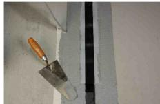
Remove the masking tape on both sides before the adhesive cures in order to achieve a clean finish.
