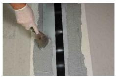
Immediately apply a second layer of adhesive on top of the tape and overlapping the tape on the sides.
