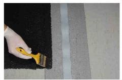
After KÖSTER KB-Pox Adhesive has cured for 24 hours, the water-proofing material can be applied overlaping onto the epoxy layer.
