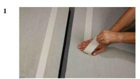
Mask both sides of the joint with tape.
