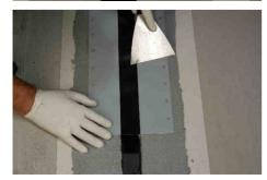
Press the KÖSTER Joint Tape onto fresh adhesive layer.
